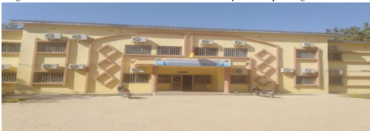
Image 1 : Exterior facade of the R+1 administrative block of the Lycée technique bilingue de Maroua
