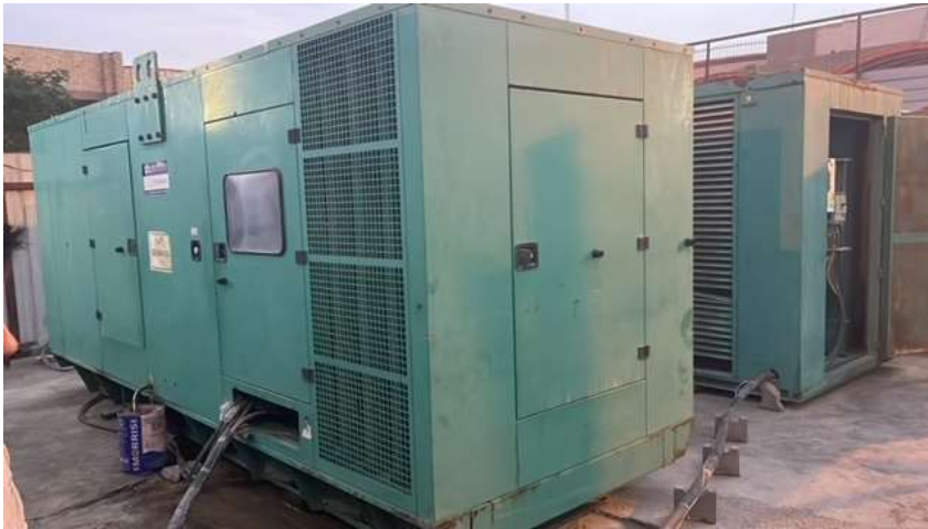
Fig. 5. Power Generators considered in this study of Perkins/Cummins generator with Power Rating of 550 KVA
